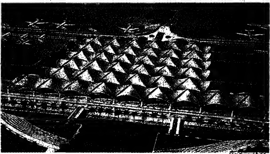
Main Terminal Building
